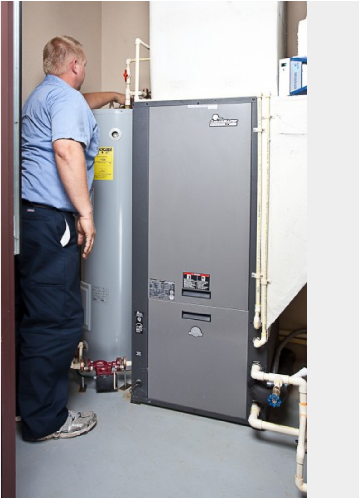
A technician inspects a geothermal HVAC air handler. Photo courtesy of Jay Egg
