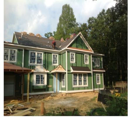
Energy House Five is moving forward quickly. With the framing being finished, siding is about to start and the insulation is being installed, some exciting things are to be reported about how this project is different from most of the homes being built today. This ENERGY STAR home is a perfect example of advanced framing standards that are helping to make this project one of the most energy efficient homes in the Alexandria community.
