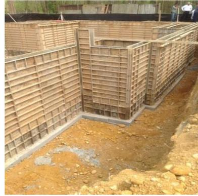
The actual pouring of the concrete on Energy House Five was done by Federal Contracting with a concrete pump truck rather than just being poured by a cement truck. This ensured that the pour was perfect with the proper amount of compacted concrete reaching corners of the foundation so no fissures or cracks occurred once the forms were stripped and removed. It was done excellently by Federal Contracting and their subcontractors.
